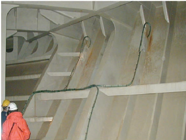
Images courtesy Light Structures
