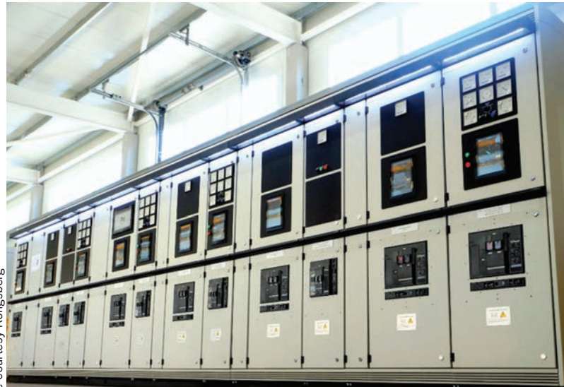
LOW VOLTAGE SWITCHBOARD
