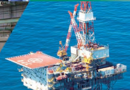
GPB30 for offshore platform
