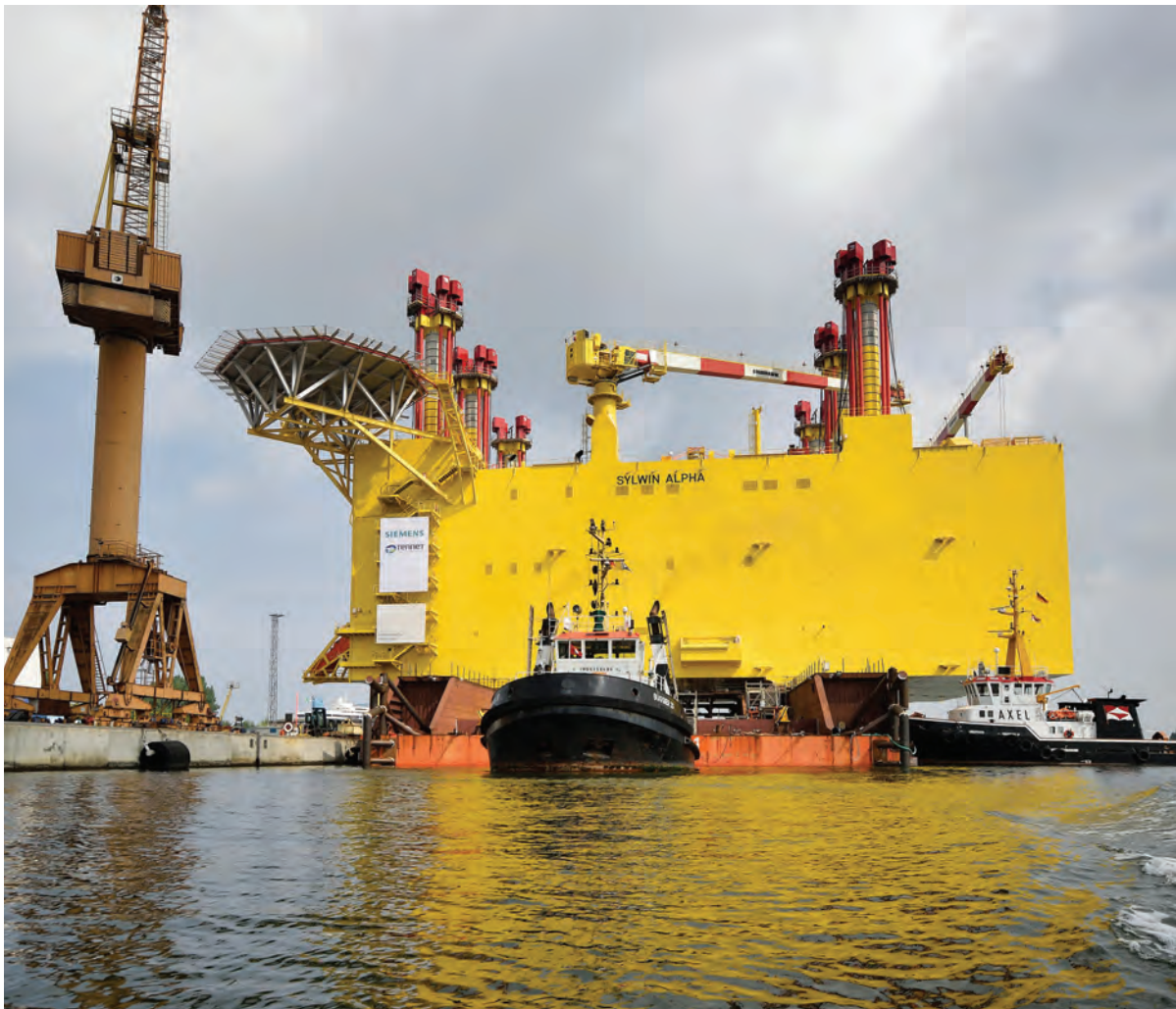
The very first transformer platform, SylWin Alpha, delivered by Nordic Yards for offshore wind energy has been installed.
