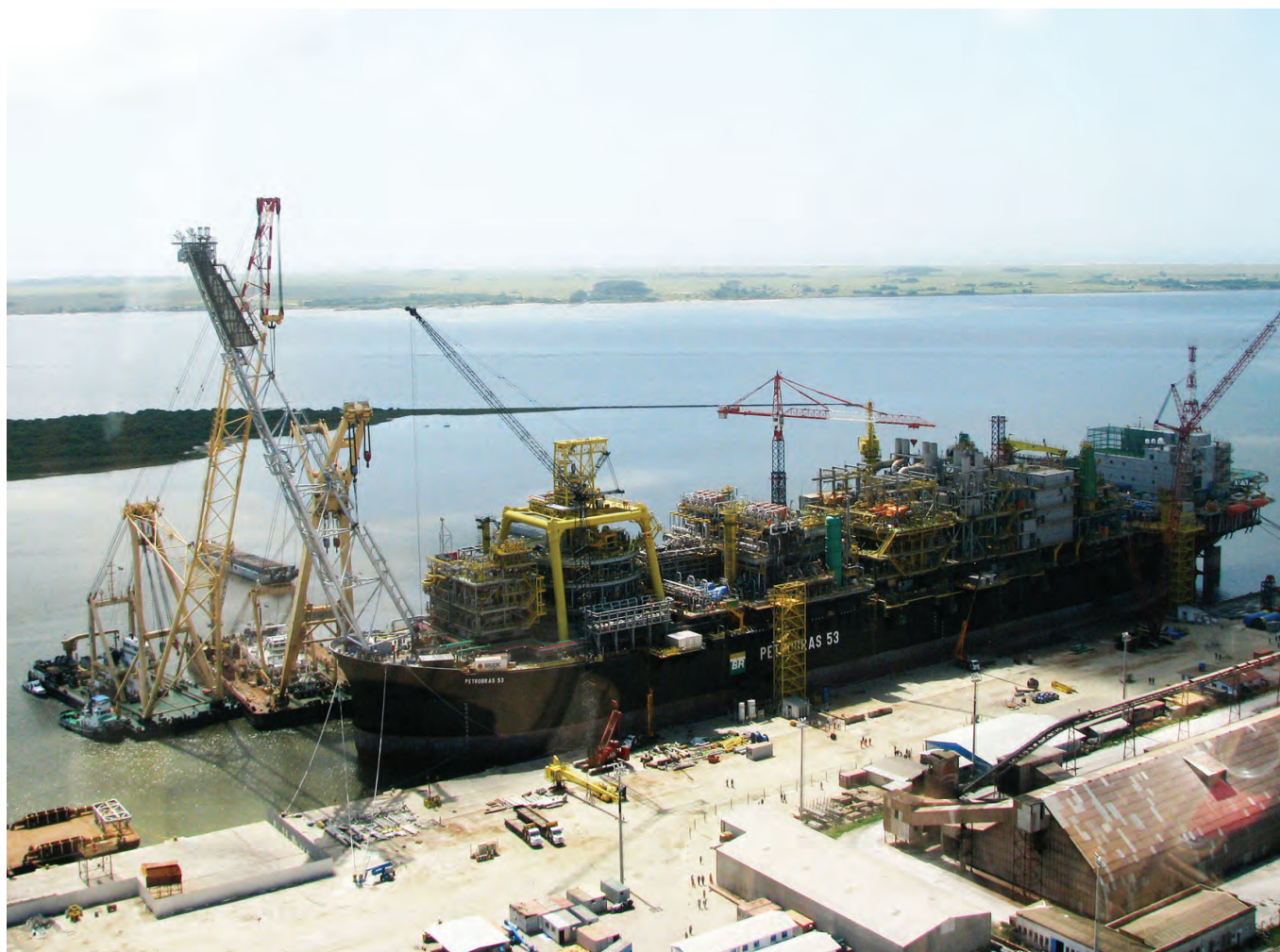
P-53 undergoing repairs and conversion.
