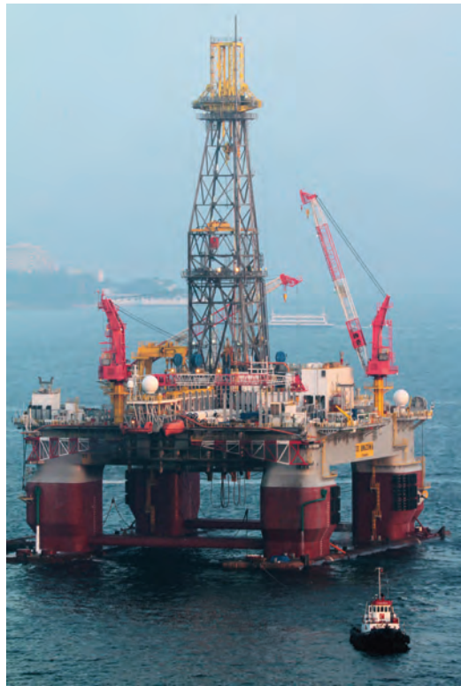
With hundreds of rigs operating offshore, specialized repair facilities are vital to the long-term viability of the current maritime and offshore energy run in Brazil.
