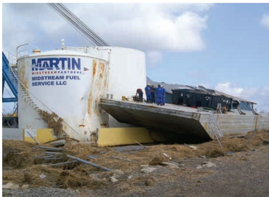
Crew working with T&T's 650-ton Big-T inspect a barge inventively displaced by Katrina's surge — the water is on the opposite side of the tank — and discover the tank is not empty. Donjon's Chesapeake 1000 was called in to minimize risk, and did the honors two days later.
