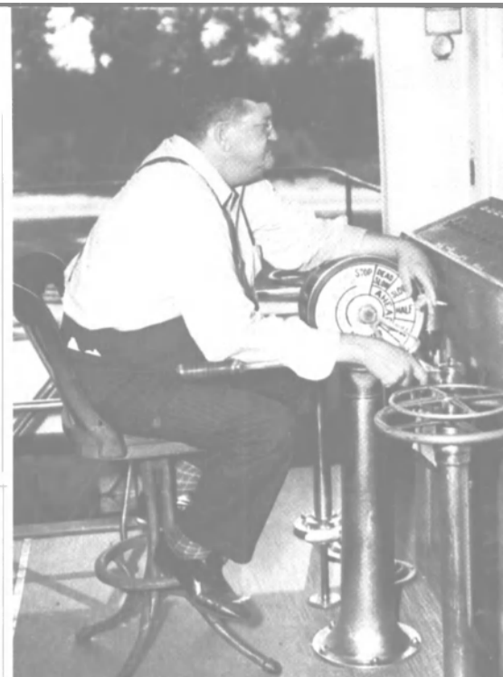
TOP: Captain Edgar "Jocko" Meeks uses a telegraph to communicate with the engine room. Pilot house control and radar navigation was not established until the 1940s. BELOW: A contemporary pilot house outfitted with advanced radar systems, computers, phones and other innovative equipment.
