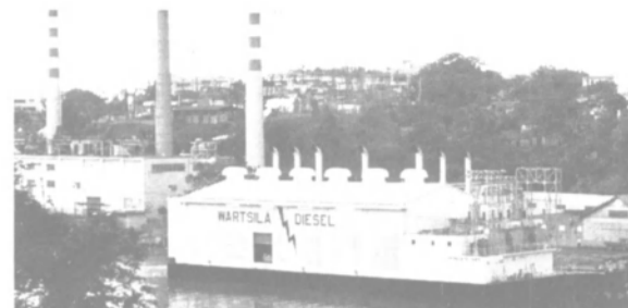
The completed barge operating on the Ozama River, Santo Domingo.
