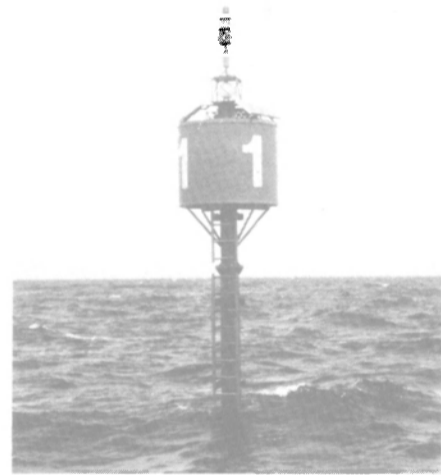
Tideland's Sentinel SAB-12 provides a stable, striking visual target for ships entering a large offshore oil port on Gulf of Mexico.
