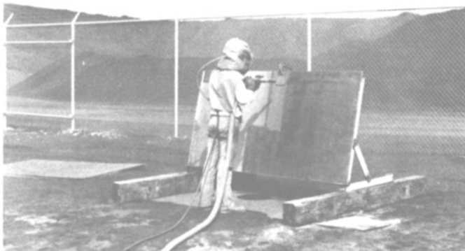
COPPER BLAST (in use here) has very little dust, is low in free silica, cuts 30-50% better than lower-quality slag abrasives and up to four times better than many silica sands.
