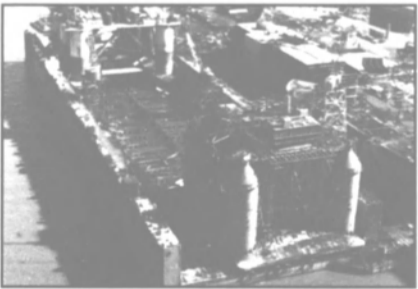
2 rigs in 900-foot length, 220-foot width inside wing walls of dock.
