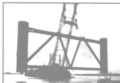
600-ton heavy lift services.
