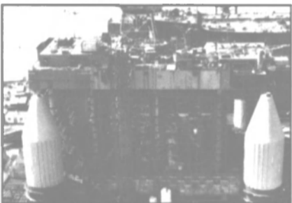
Structure erected, return to dock.
