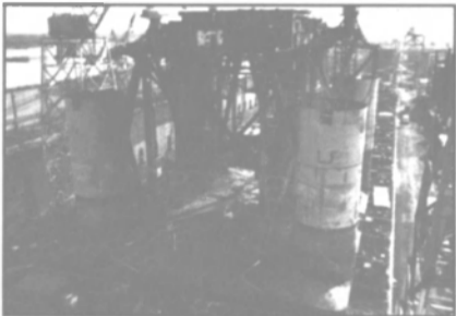
Column removal, deckhouse rebuilding.
