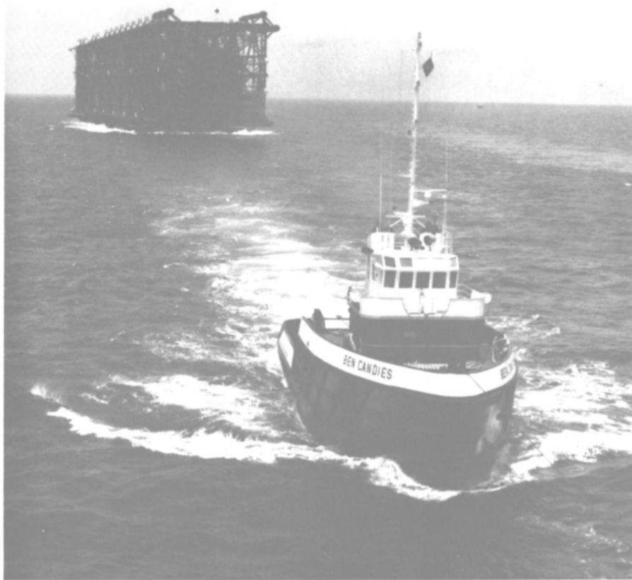
The Ben Candies, powered by two EMD 16-645-E6 main diesel engines, shown towing the first guyed tower platform installed in Gulf of Mexico.
