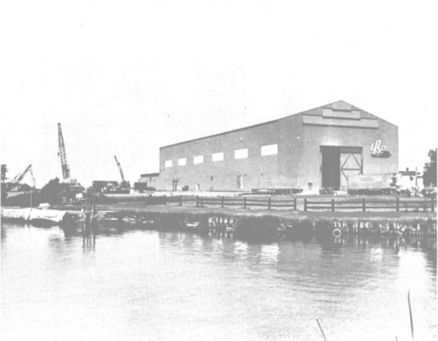
View of fabrication building and yard cranes from across the Ontonagon River.
