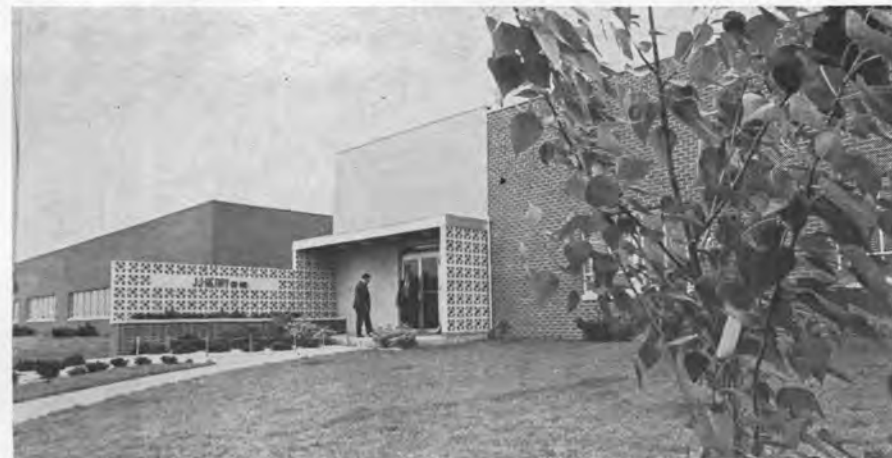
NEW HEADQUARTERS for the Philadelphia office of the J.J. Henry Co., located in an industrial park in suburban Moorestown, N.J., is a one-story air-conditioned building.
