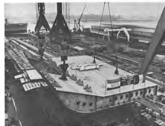
FIRST EUROPEAN-BUILT LASH: Construction of the first two LASH (Lighter Aboard Ship) vessels to be built in Europe is under way at the Cockerill Yard, Hoboken, Belgium. The keel laying for the first ship, shown above, took place on June 7. The ships, designed by Friede & Goldman, Inc., naval architects of New Orleans, La., are being built for Holland-America Line and Hapag-Lloyd Lines. Both will be operated by Combi Line, a newly-formed operating group. Delivery is scheduled for 1972. Both ships are scheduled to operate on a trade route serving U.S. Gulf and East Coast ports, and ports in Northern Europe. Their principal characteristics include overall length of 857 feet, beam of 105 feet, height of 60 feet, deadweight of 43,500 tons, with accommodations for carrying 73 standard LASH lighters and a number of 20-foot and 40-foot containers. Propulsion unit is one 26,000-hp Sulzer diesel engine. A total of 21 LASH ships, aggregating more than a half-billion dollars of shipping, are operating or on order. They will serve ports on five major world trade routes.
