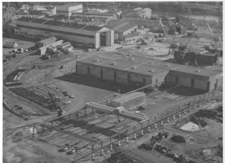
Overall view of Marine Industries Limited shipyard in Sorel, Quebec, showing in the foreground the new steel storage and painting facilities and the fabrication shop.
