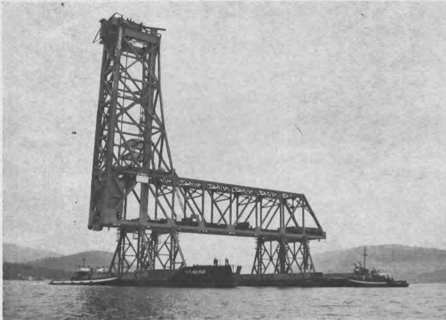
1. Vancouver Tug Boat Co. Ltd. scored a major tugboating feat in Vancouver Harbor recently as it floated the new Canadian National Railways bridge into place at 2nd Narrows in three sections. Shown above, the south tower, weighing 2,000 tons and measuring 200 feet high and 250 feet long, is being moved by Vantug.
