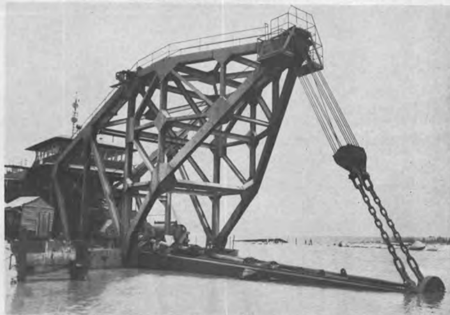
The 'working end' of the dredge Bill Bauer shows the suction ladder after installation. The ladder, weighing 350 tons, including the suction head, is made of Armco SSS 100 steel plate, with yield strength of 100,000 psi.
