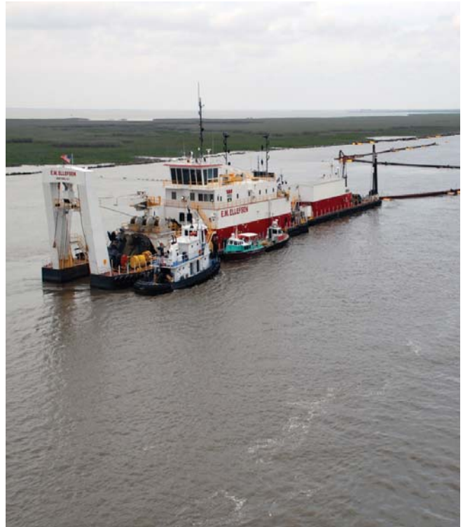
Photograph courtesy U.S. Army Corps of Engineers, New Orleans District
