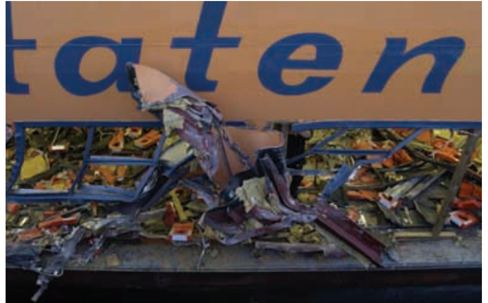
The outside lower level of the Staten Island Ferry Andrew J. Barberi after it struck a pier killing ten people October 15, 2003. USCG photo by PA2 Mike Hvozda.
