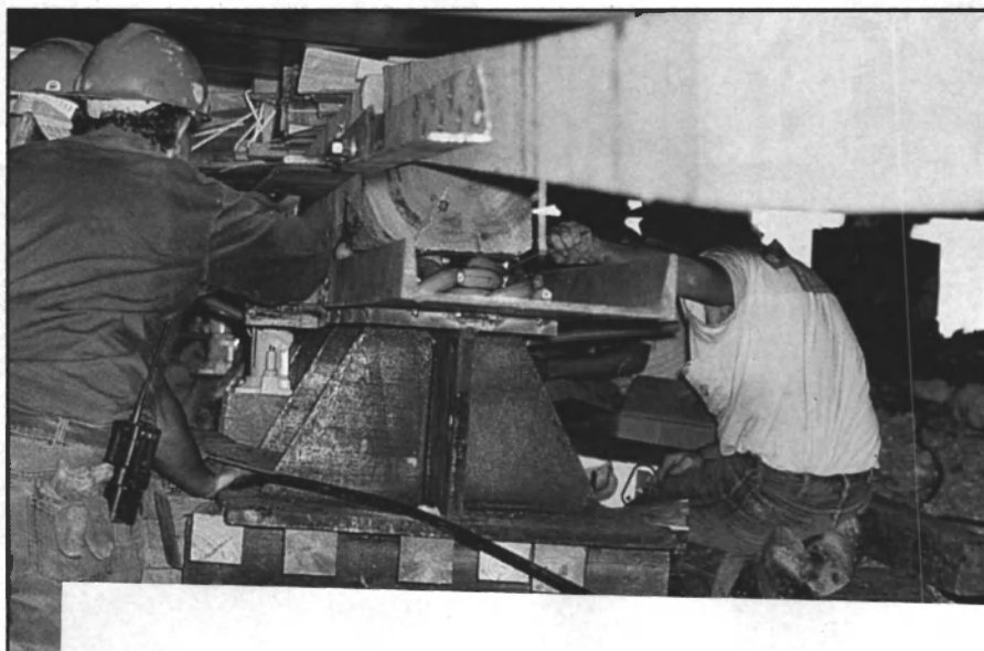
Pictured is the insertion of bananas into the slide rails of the Branson Belle by Minnesota-based company Power Team. Ten cases of the lubricant were used per slide rail during the launch.
