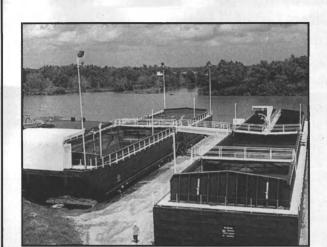
The new waste water treatment facility at Bourg Dry Dock & Service, Bourg, La., handles oil waste waters at a rate of 300 gpm
