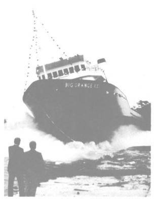
Moss Point Marine, Inc. of Escatawpa, Miss., recently launched a big towing/supply vessel for Intermarine of Houston. The vessel has an overall length of 218 feet, beam of 40 feet, and depth of 14 feet. It was named the Big Orange XXI.
