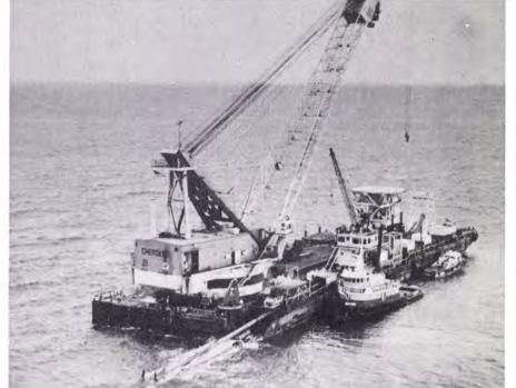
SANTA FE INTERNATIONAL'S CHEROKEE, converted to work as bury barge on Ekofisk pipeline, has eight 4,000 BHP Alcos driving high pressure water pump to bury sled.
