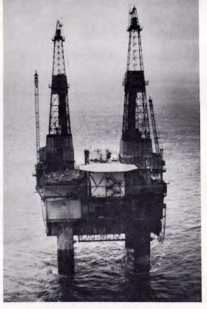
This production platform in Cook Inlet, Alaska, represents a complete oil field operation, including water injection field. Johnston pumps, highly suitable because of their vertical configuration, serve as crude oil loading pumps.
