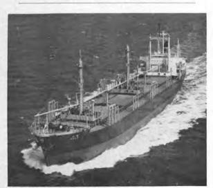
LOG/BULK CARRIER HALO, which was built at Hitachi Zasen's Innoshima shipyard, has been delivered to her owner, Liberian Halo Transports, Inc. The 564-foot 4-inch vessel is built to the shipyard's economical standard design with sufficient stability for deck loading of logs. The 23,547-dwt ship is propelled by a Hitachi B&W 762-VT2BF-140 diesel engine developing 8,400 bhp and giving the ship a service speed of 14.5 knots.
