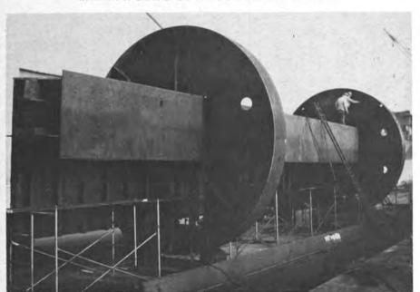
Special rolling rings hold box girder and position it for down-hand welding.
