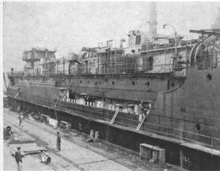
Stripping off the sheer strake and preparing the hull to receive the prefabricated box girder before gutting the ship. No strapping of the hull is necessary.
