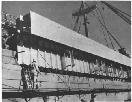
Installing a new box girder section which forms part of the shell and longitudinal bulkhead and the deck on one side. The deck level is raised two feet.
