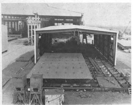
Motorized buildings equipped with plant services enable workmen to subassemble sections under ideal conditions.
