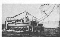
The Imodco SPM system provides a simple, economical solution to the problem of loading and discharging supertankers and other bulk liquid carriers which have already outgrown all but a handful of the world's existing port facilities. Securely anchored offshore, it permits cargo operations to continue under nearly all weather and sea conditions. Floating hoses, which
